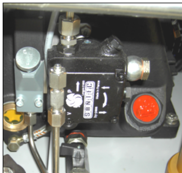
Oil Pressure Switch & Oil Pump
